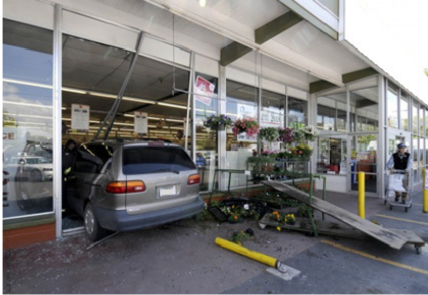
Figure 4: Vehicle Crashes through Bollard into Grocery Store
